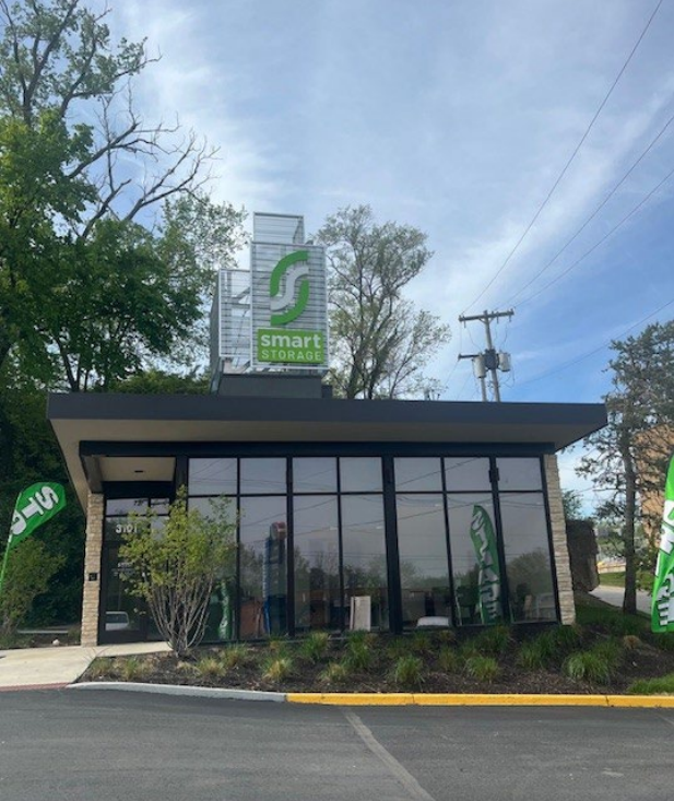
View of the Smart Storage office and 3101 elevator to Downtown Underground looking south from 31 st Street and Mercier
