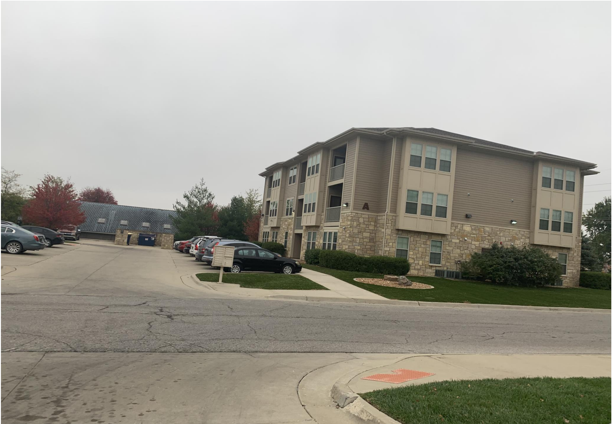
5. EXTERIOR OVERVIEW- BUILDING A
