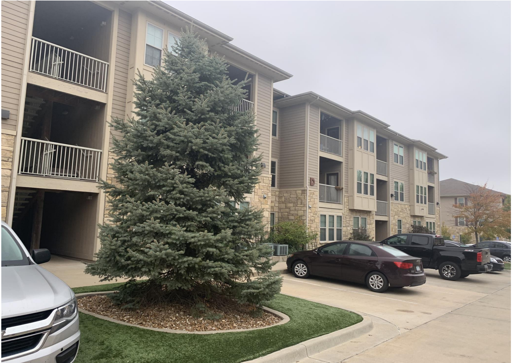
16. EXTERIOR OVERVIEW- BUILDING D
