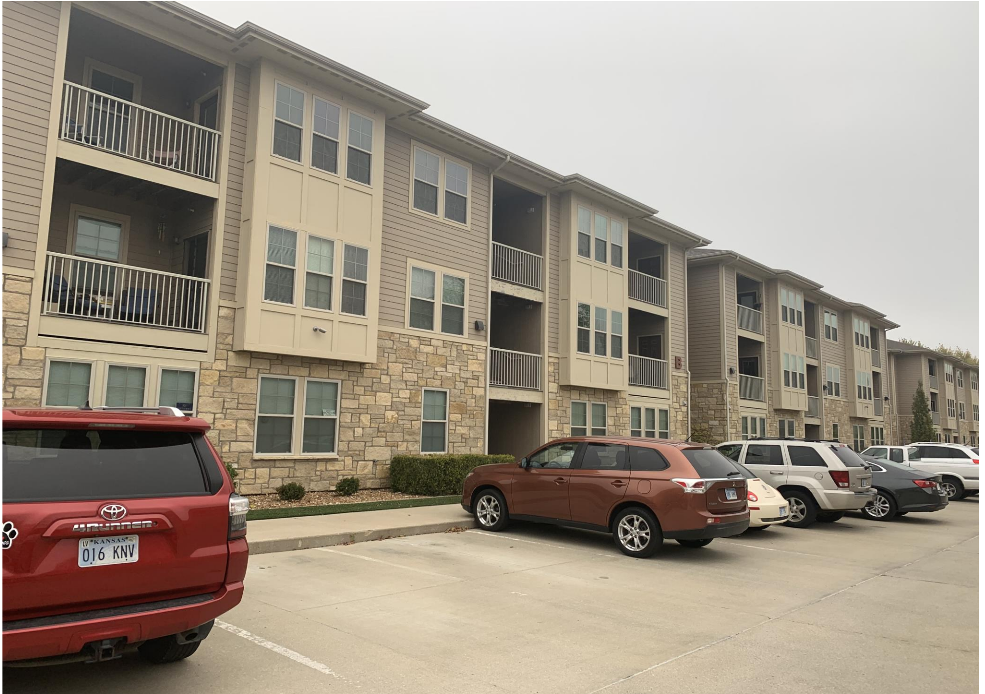
9. EXTERIOR OVERVIEW- BUILDING B
