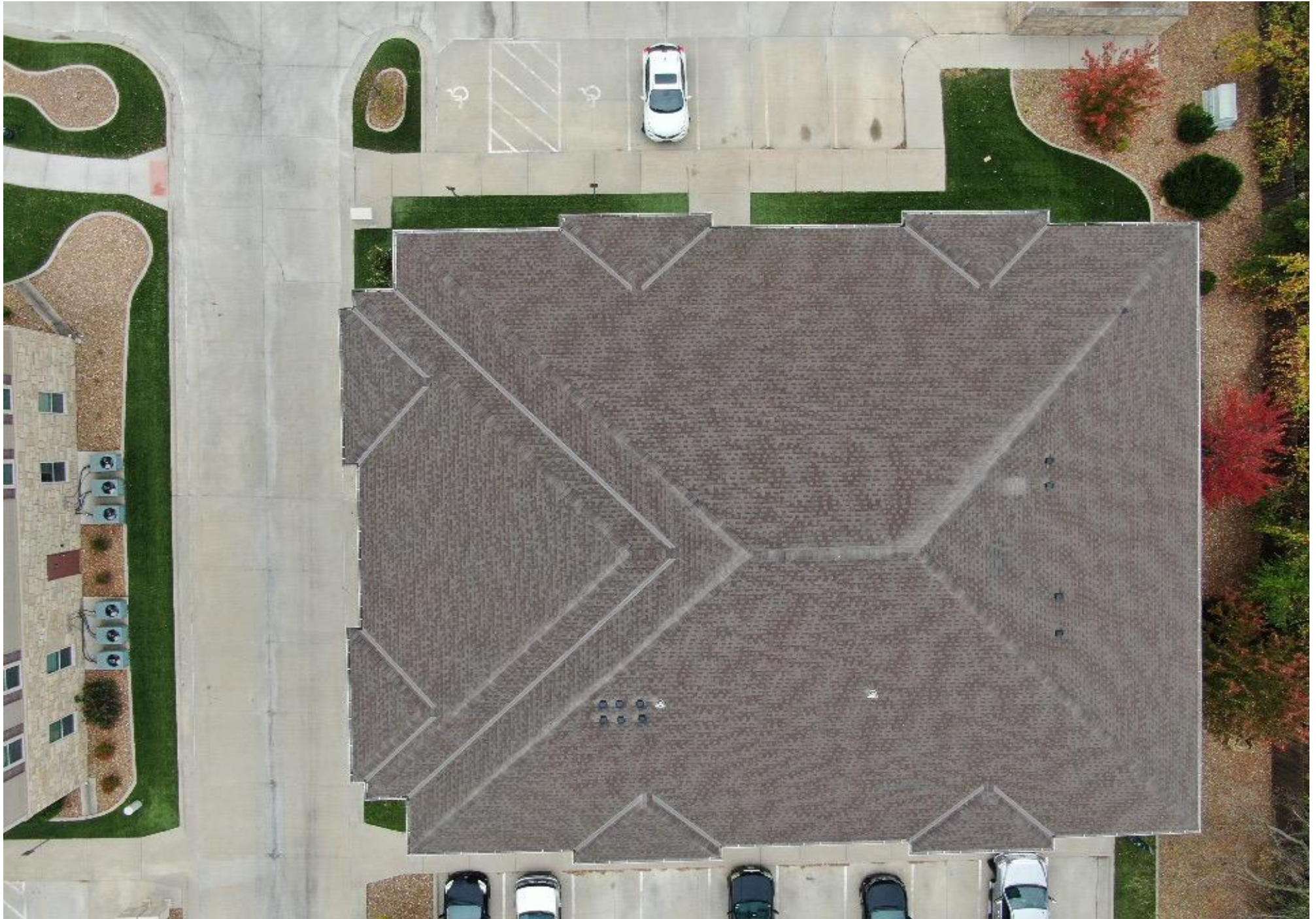
15. ROOF AREA OVERVIEW-BUILDING C
