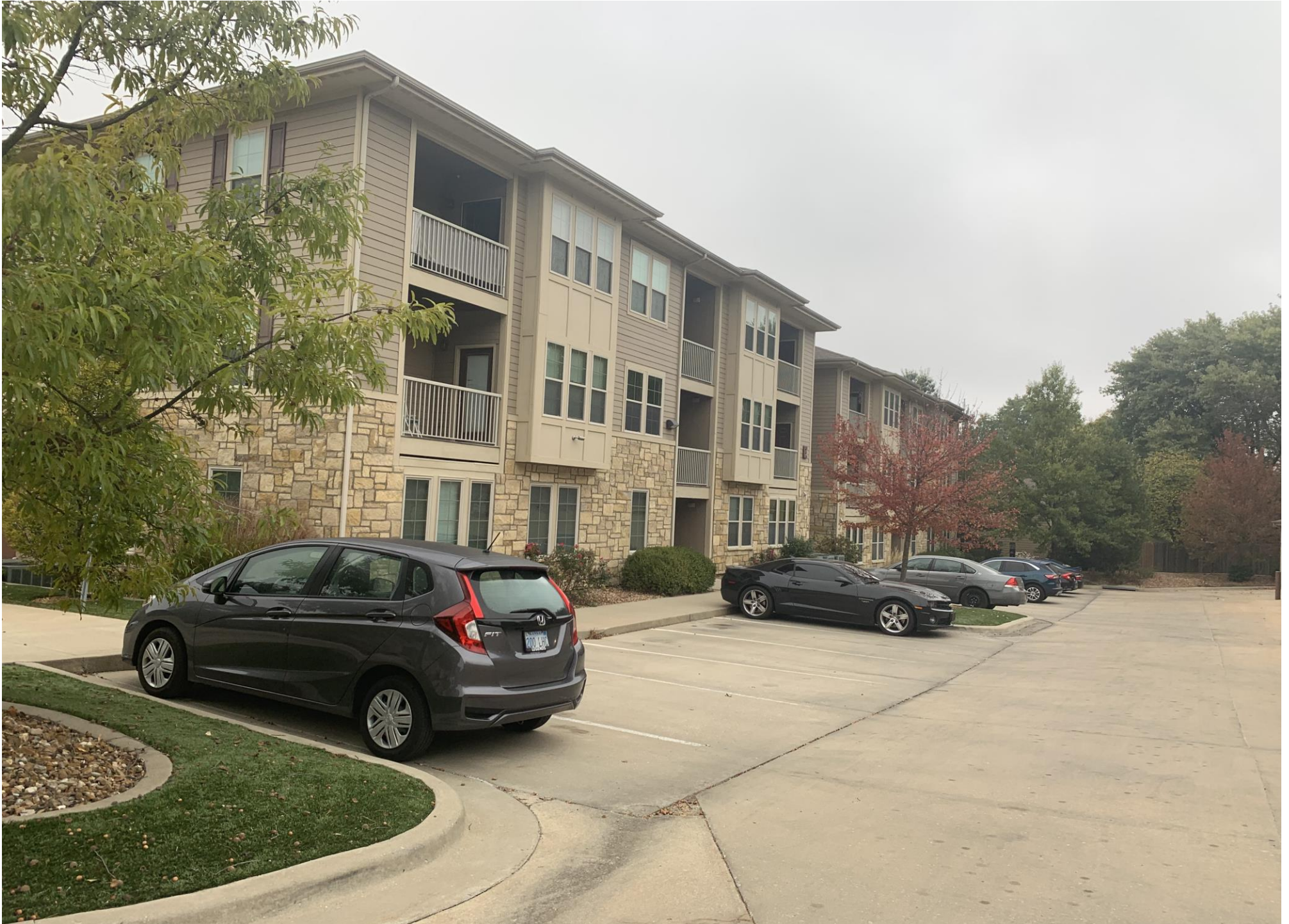
22. EXTERIOR OVERVIEW- BUILDING E
