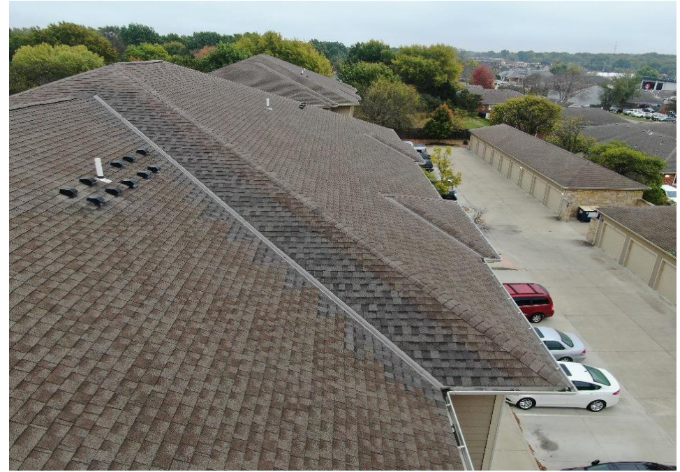
12. OVERVIEW OF PAST VALLEY SHINGLE REPLACEMENT
