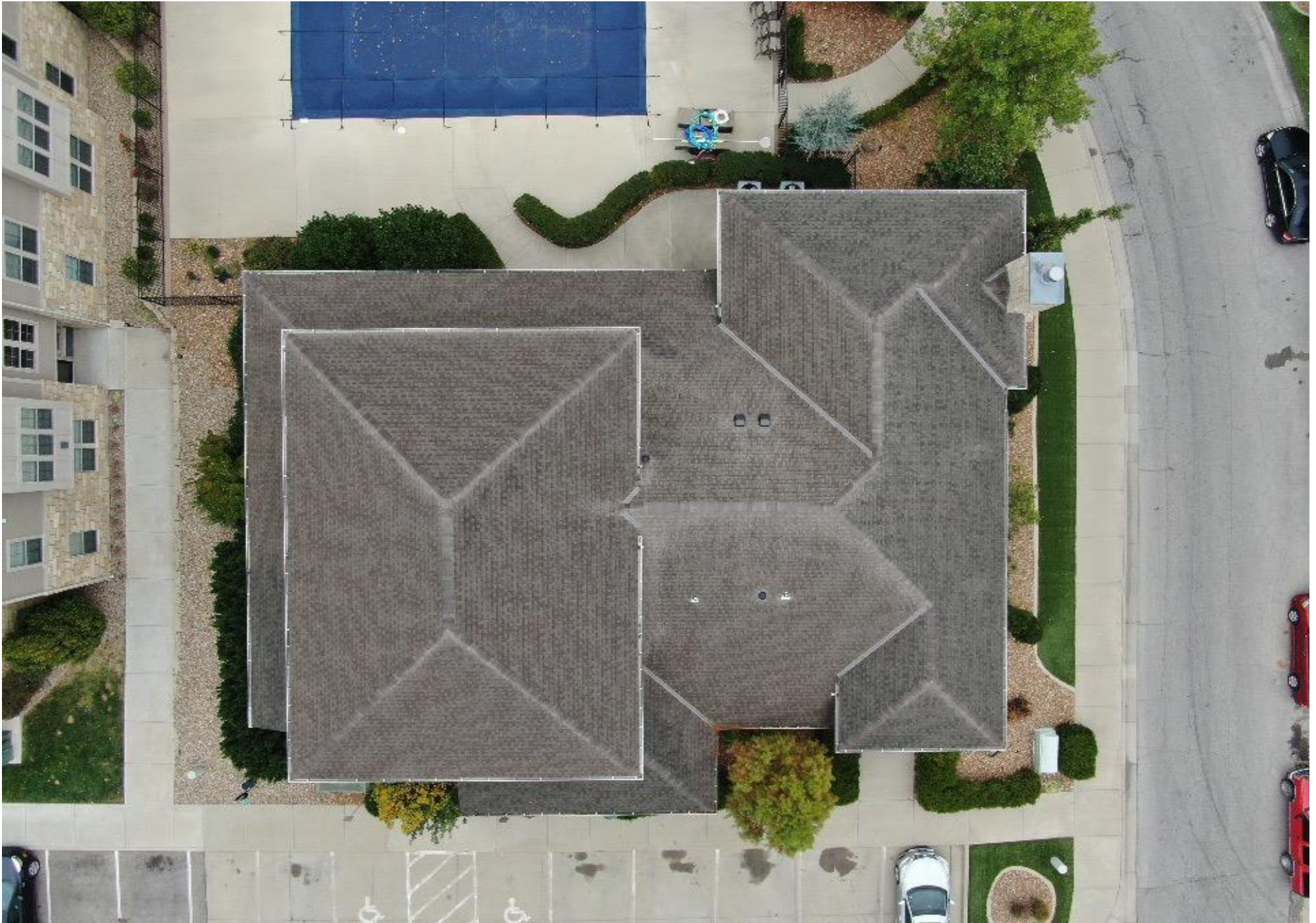
33. ROOF AREA OVERVIEW-CLUBHOUSE BUILDING
