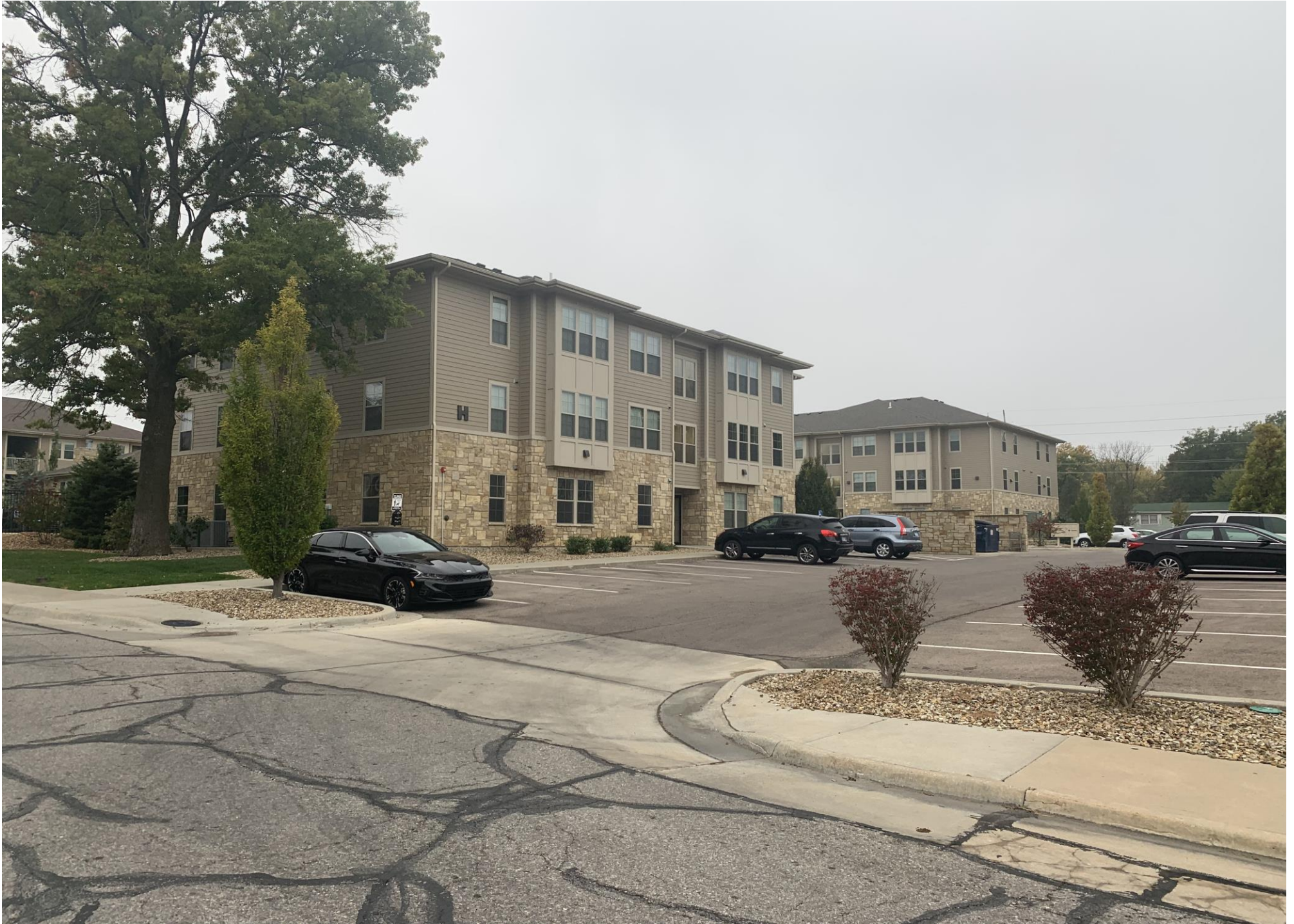
29. EXTERIOR OVERVIEW- BUILDING H
