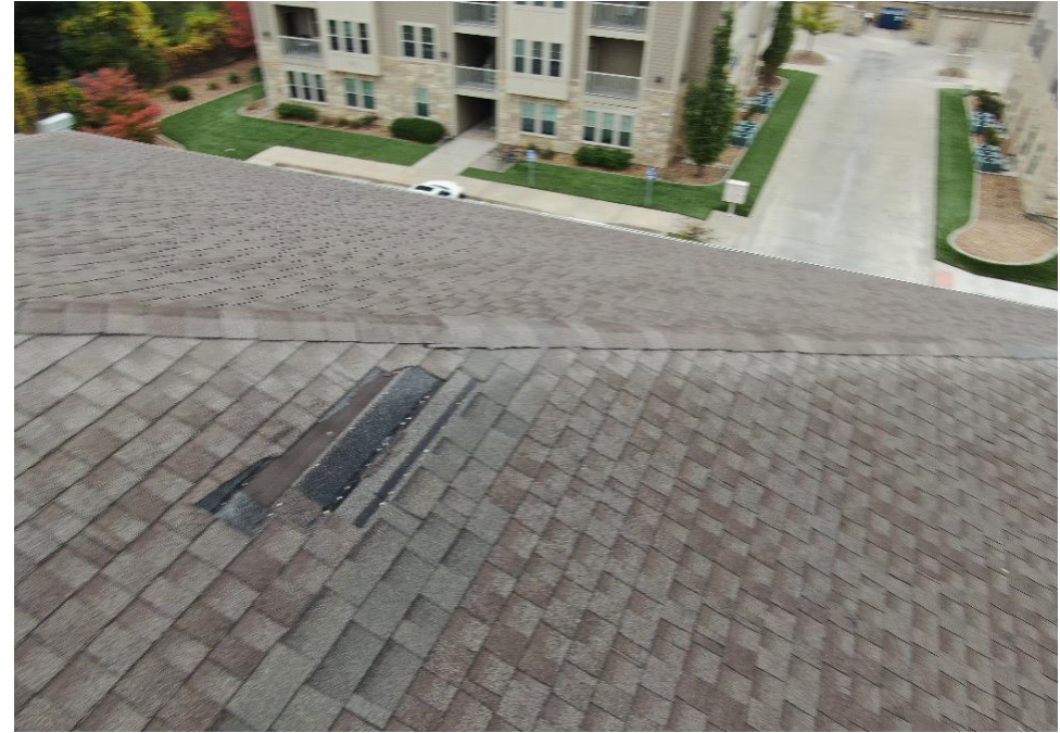
19. MISSING SHINGLES
