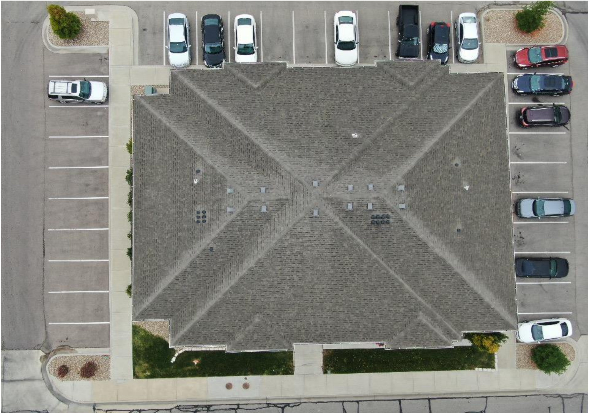
37. ROOF AREA OVERVIEW-BUILDING J
