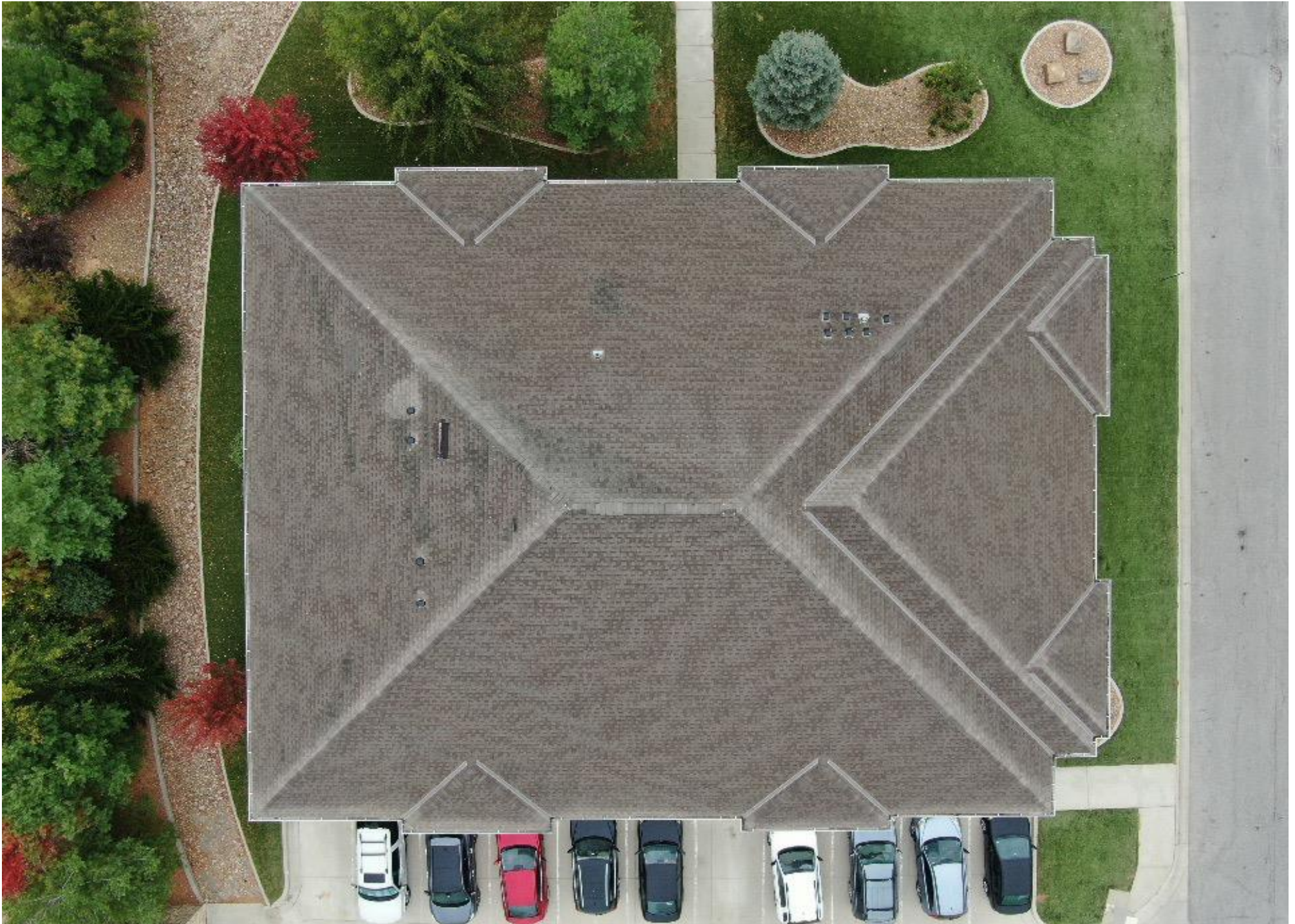
6. ROOF AREA OVERVIEW-BUILDING A
