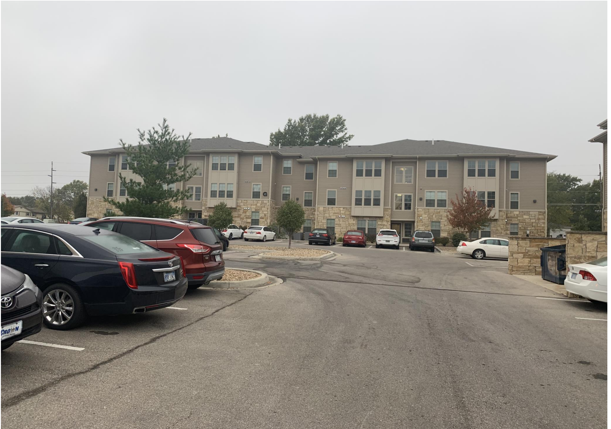
27. EXTERIOR OVERVIEW- BUILDING G
