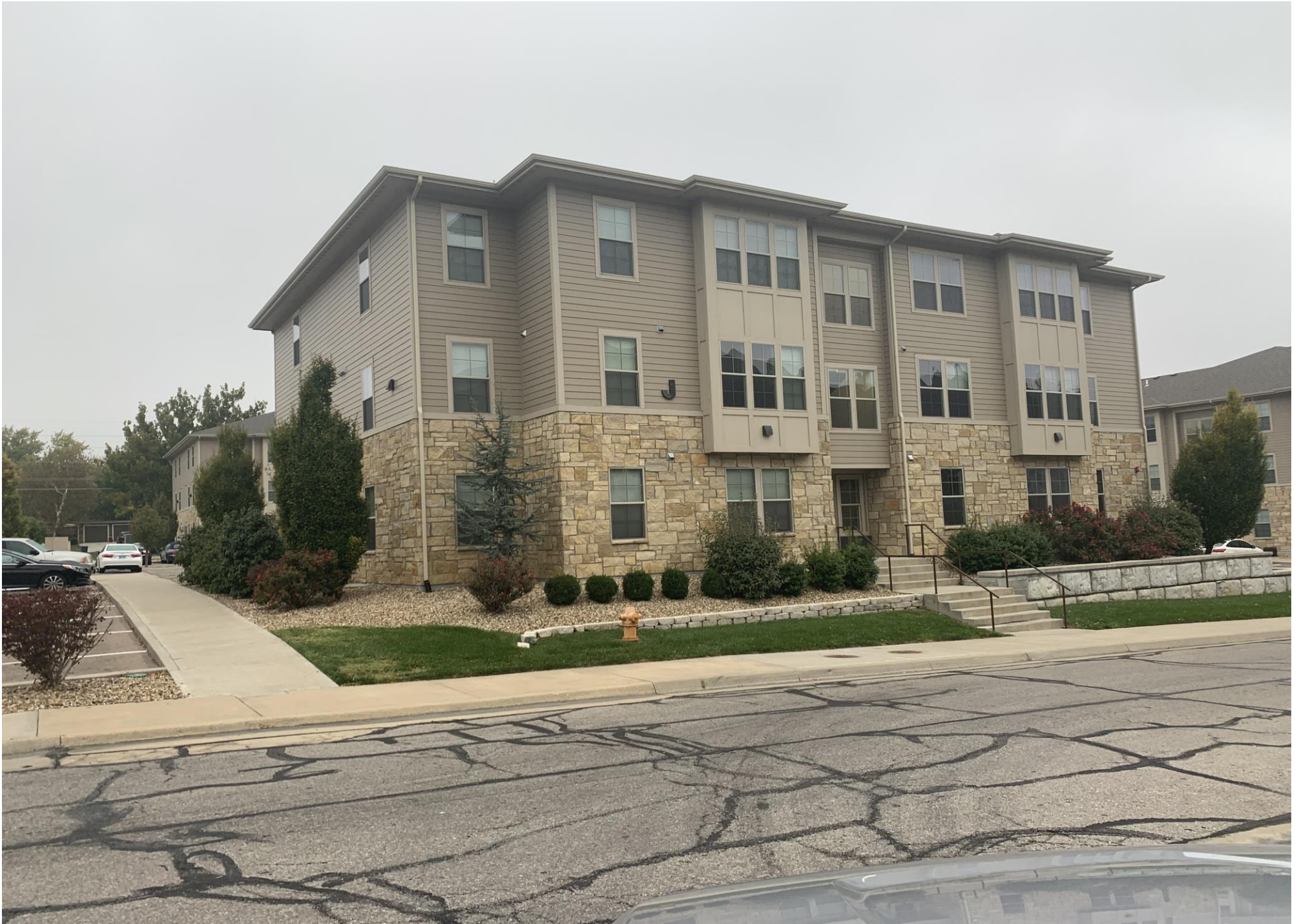
36. EXTERIOR OVERVIEW- BUILDING J
