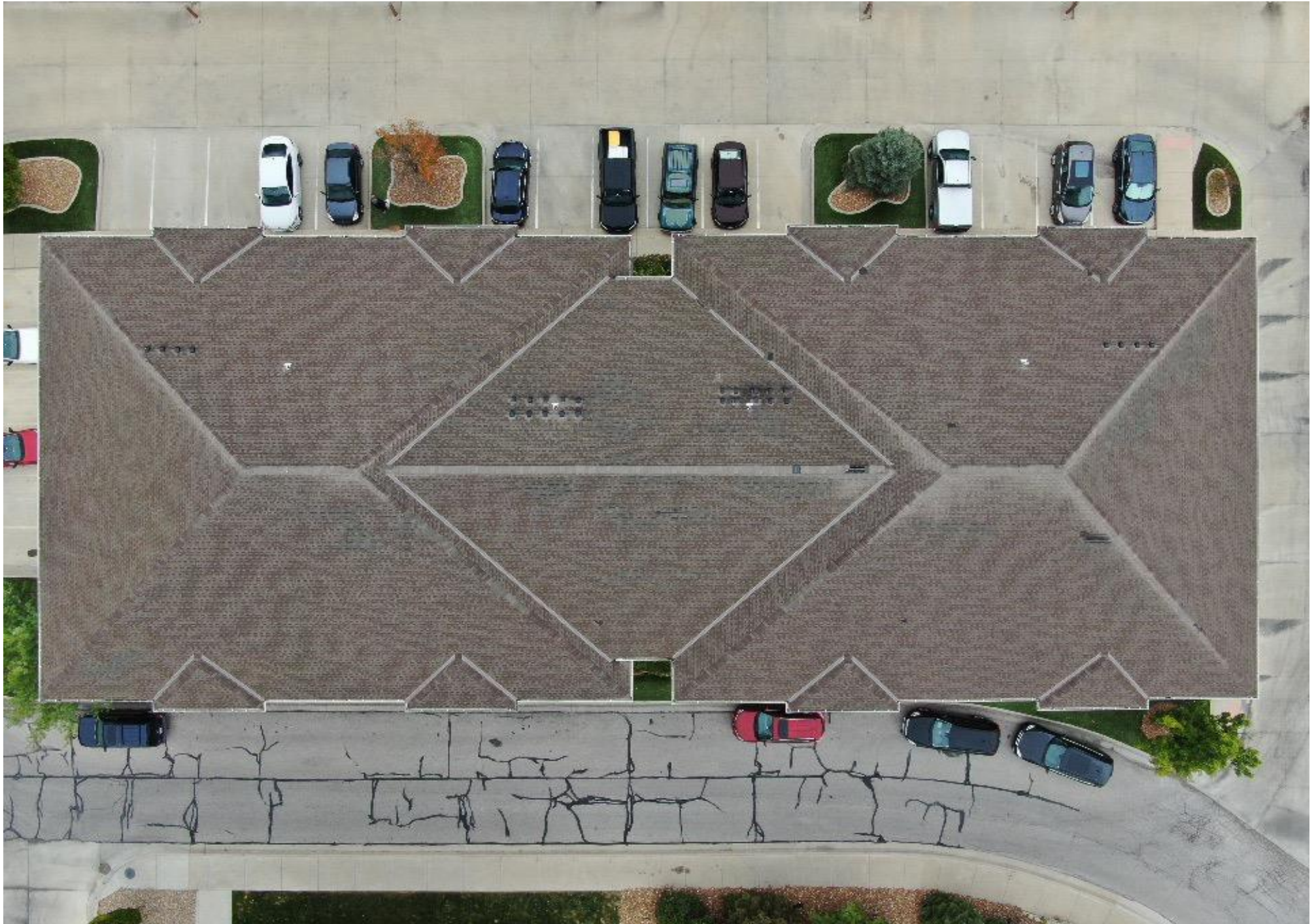
17. EXTERIOR OVERVIEW- BUILDING D
