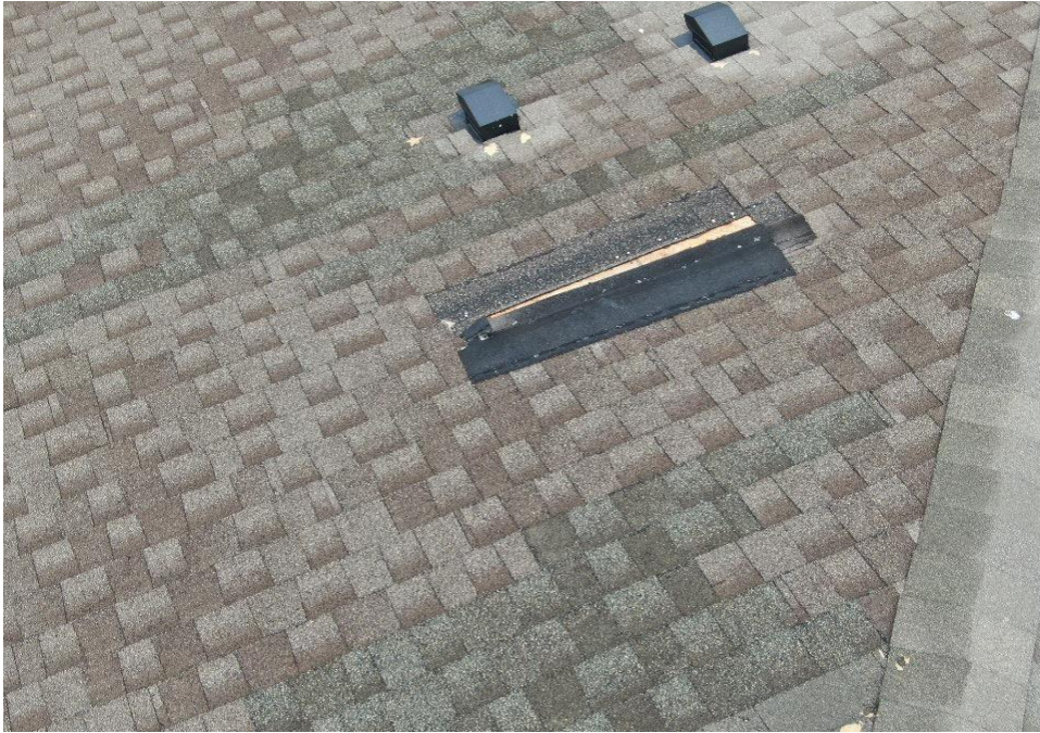
7. LOOSE/MISSING SHINGLE
