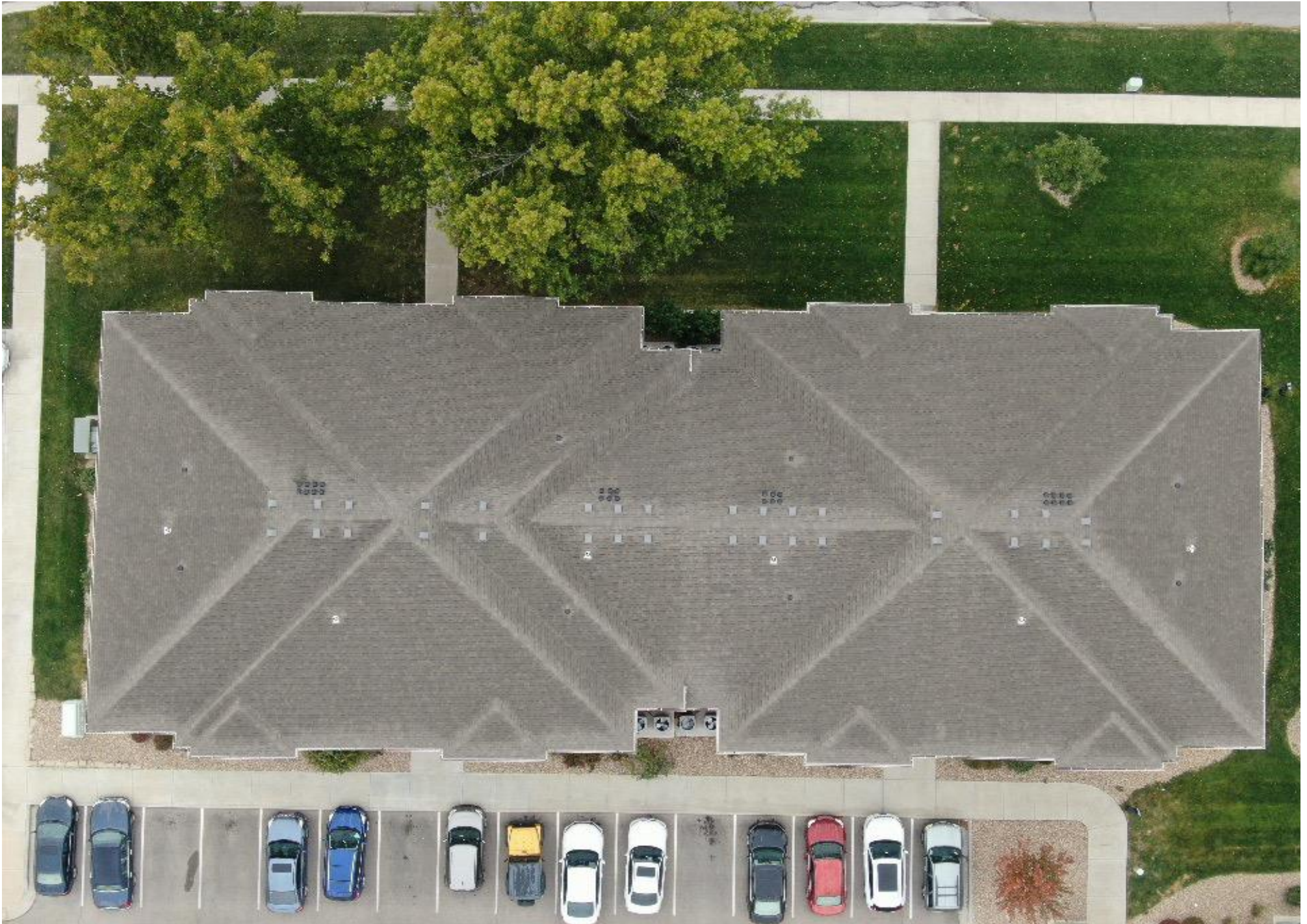
28. ROOF AREA OVERVIEW- BUILDING G
