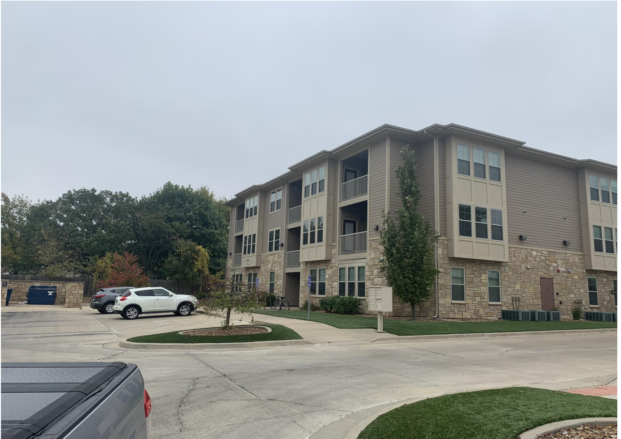
14. EXTERIOR OVERVIEW- BUILDING C
