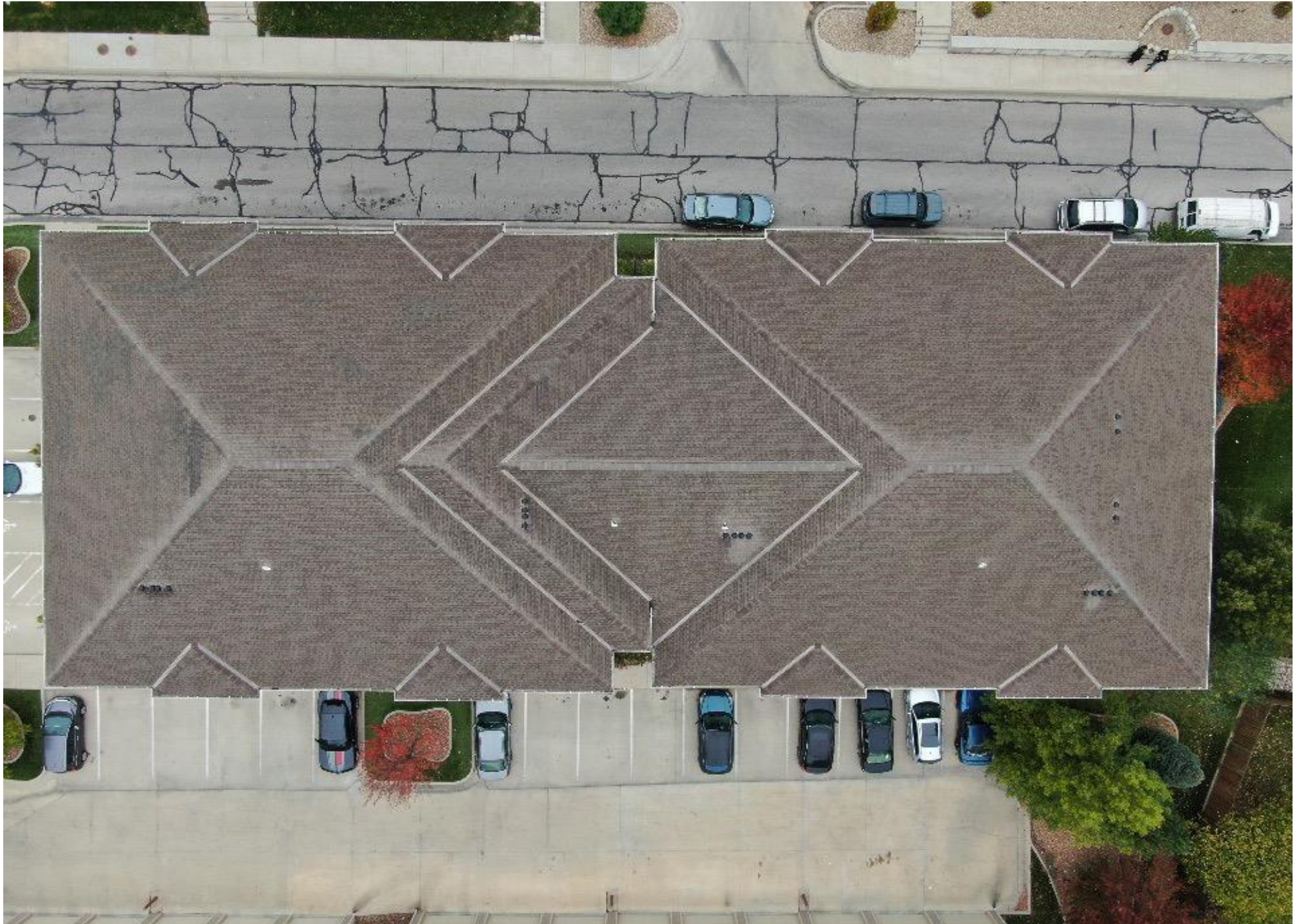
23. ROOF AREA OVERVIEW-BUILDING E
