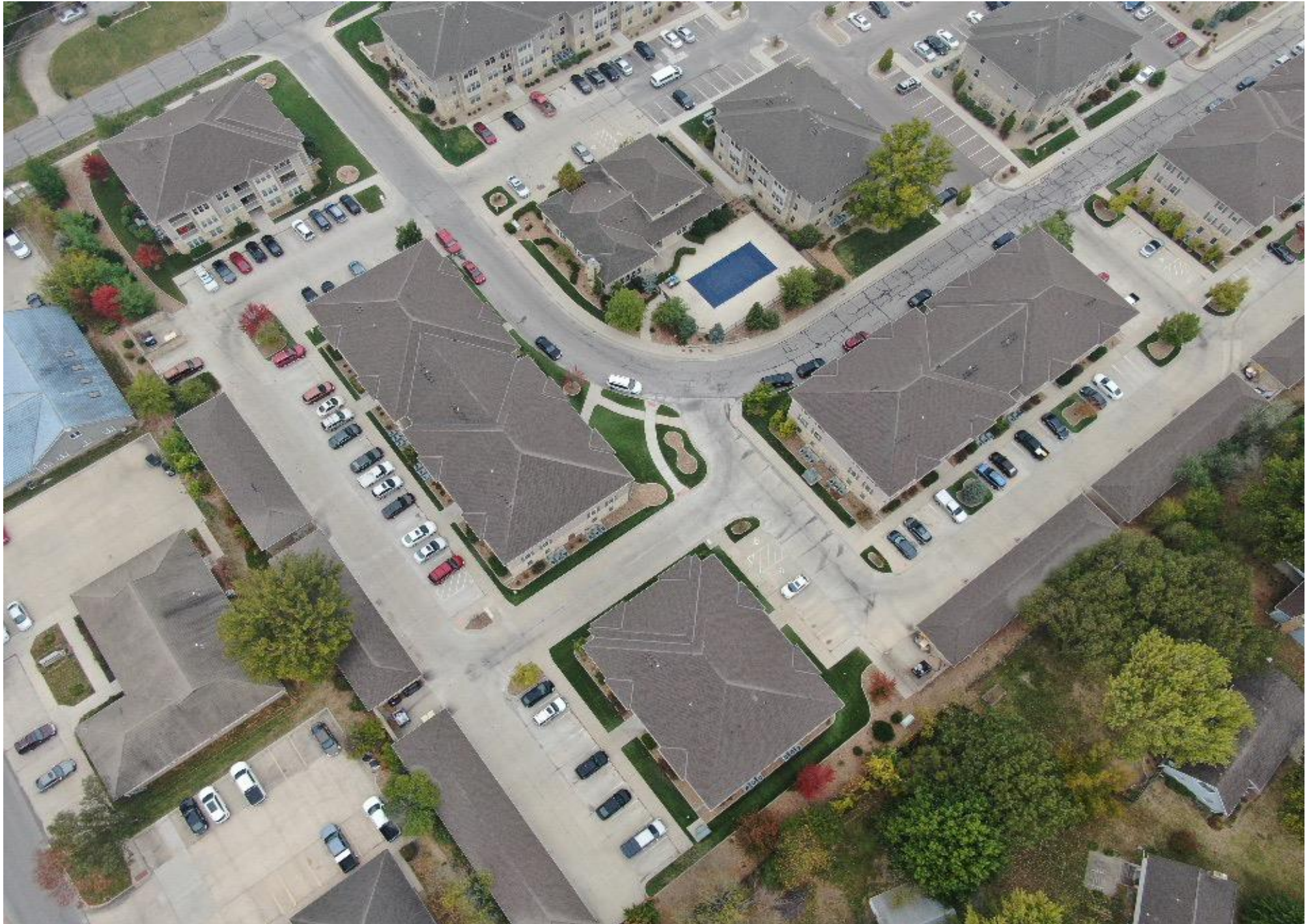
3. AERIAL OVERVIEW OF PROJECT SITE
