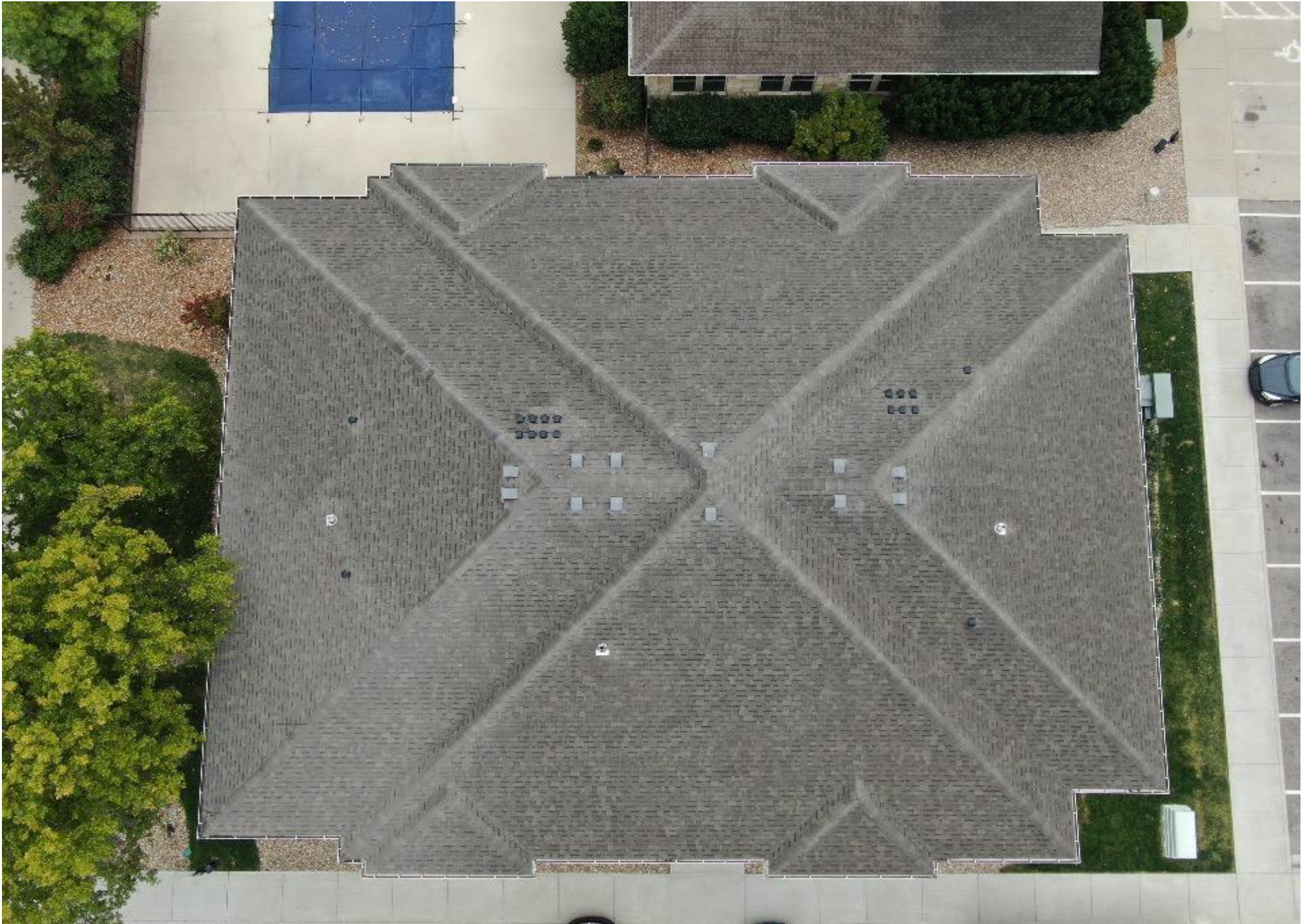
30. ROOF AREA OVERVIEW-BUILDING H
