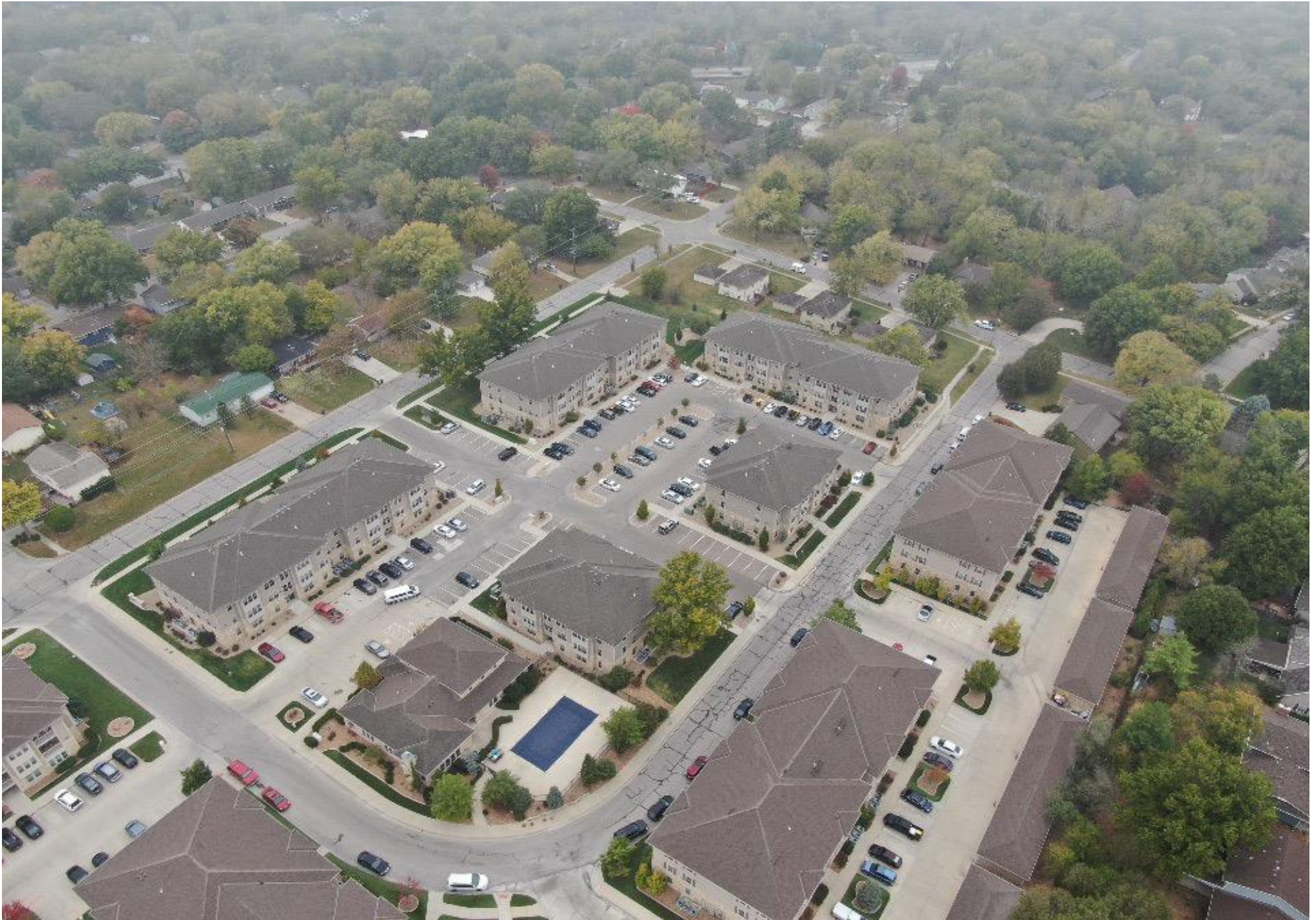
4. AERIAL OVERVIEW OF PROJECT SITE
